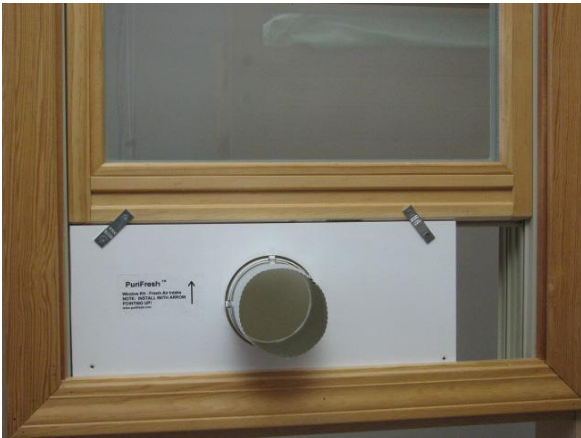
Figure 3: Attach the Fresh Air Intake to the window sash using the mending plates and flat head wood screws, as shown. BE SURE THAT THE ARROW IS FACING UP.
